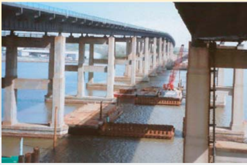
Design/Build New Route 9 Bridge over Raritan River, Edison, NJ Owner: NJ Dept. of Transportation Construction Engineering
