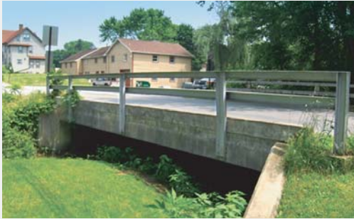
Design/Build Irish Creek Road Bridge, Centerport, PA Owner: Pennsylvania Dept. of Transportation Superstructure Replacement and Roadway Design Traffic Control, Right-of-Way and Permitting
