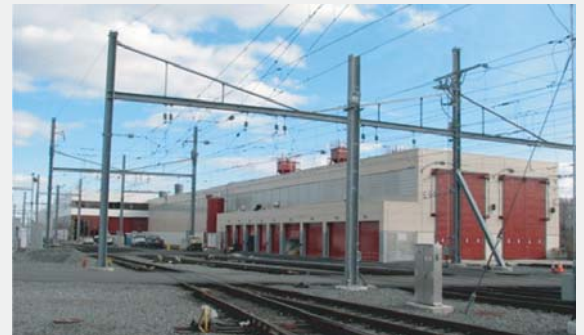
Design/Bid/Build Morrisville Train Storage Yard (Phase 2), Morrisville, PA Owner: NJ Transit Corporation Site / Civil and Geotechnical Engineering
