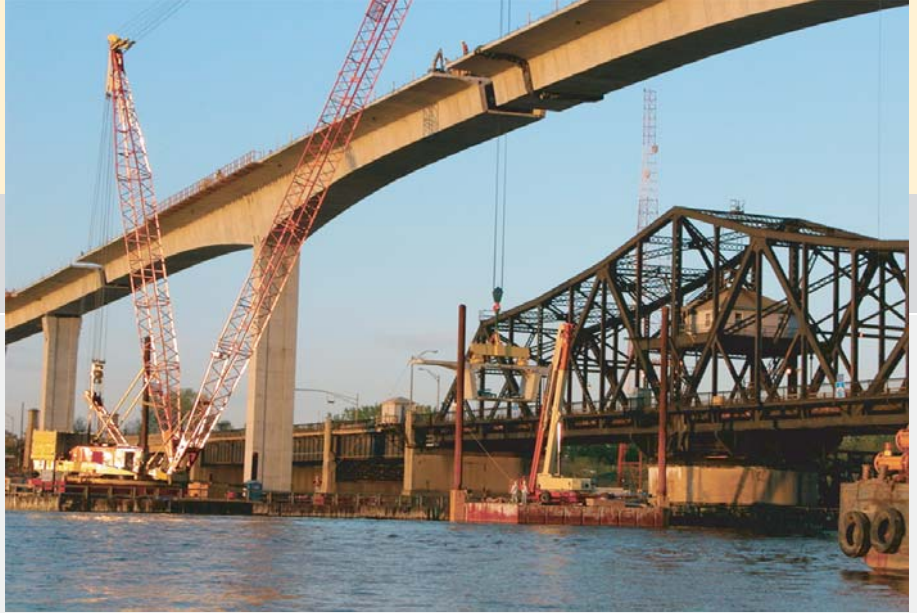
Design/Build New Route 35 (Victory Bridge) over Raritan River, Rahway, NJ Owner: NJ Dept. of Transportation Construction Supervision
