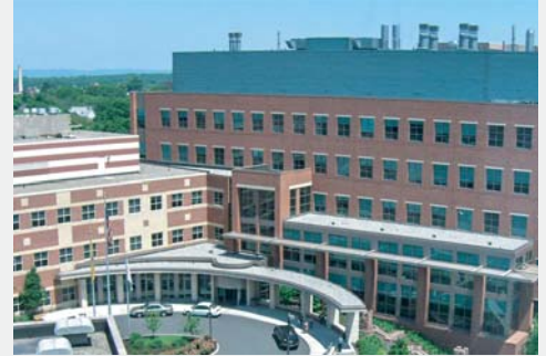
Design/Build Renovation of Robert Wood Johnson Medical School New Brunswick, NJ Owner: University of Medicine and Dentistry of NJ Structural Engineering
