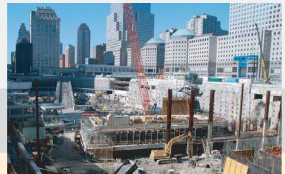
Design/Build PATH World Trade Center Transportation Hub Owner: Port Authority of NY & NJ Structural Engineering during Construction
