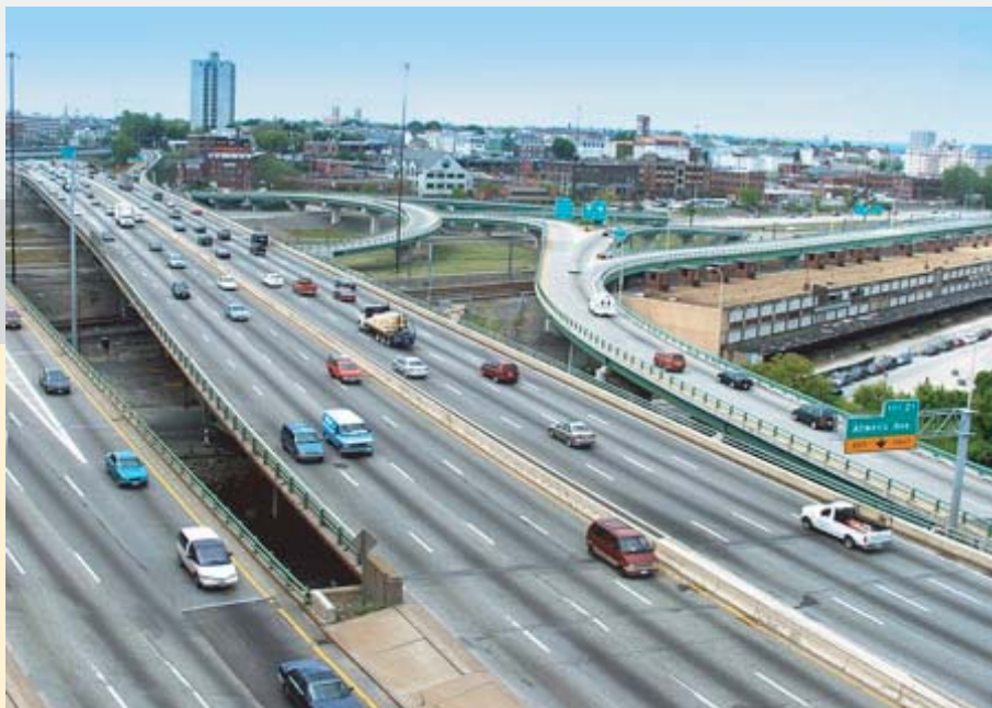
Design/Build I-95 Providence Viaduct, Providence, Rhode Island Owner: Rhode Island Department of Transportation Engineering Support for Construction Sequence
