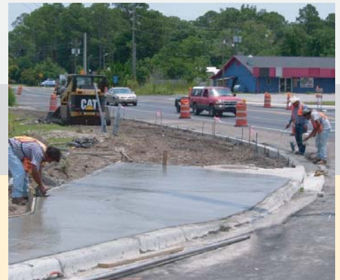
Design/Bid/Build Sidewalk & ADA Ramps, NY City Owner: NYC Dept. of Design & Construction Construction Engineering
